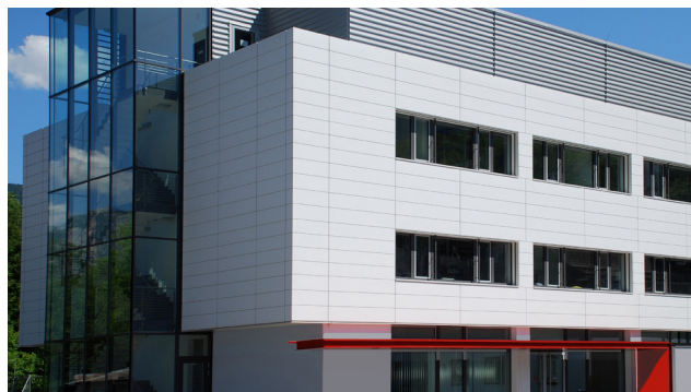
Pharmaceutical Lab Building
