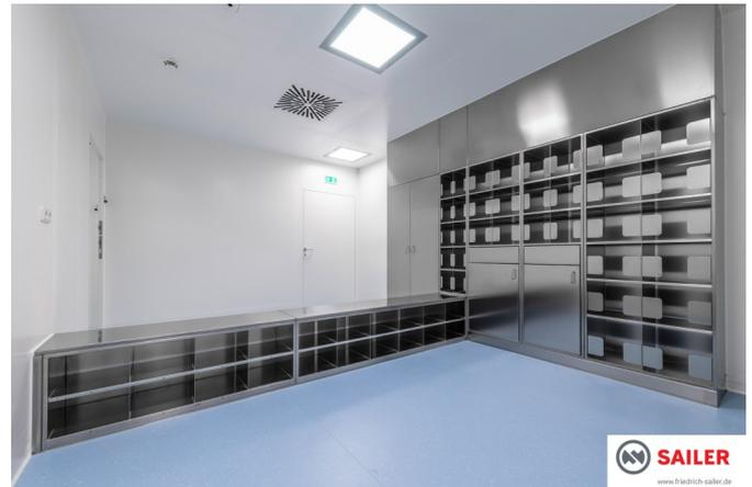
In addition to the work rooms, Friedrich Sailer GmbH was also responsible for the design and implementation of the personnel airlocks. HPL materials were used in the airlocks between CNC/D and D/C, while for the airlocks between classes C and B the choice fell on airlock equipment made entirely of stainless steel.
