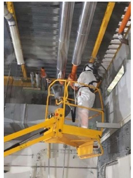
At the start of dismantling operations, CURIUM and Jobbing's teams first inerted the networks with nitrogen to avoid explosion risk, then unbridled or cut within glove bags the sections to be deposited. The sections were then dedusted, reduced in size according to the waste treatment facility's specifications, and packaged in compliance with hazardous goods transportation regulations.
