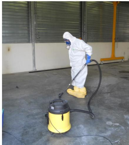
CURIUM's specialists began with a thorough contamination analysis in all areas and on a variety of surfaces. Contamination diagnostics is an important step before starting the decontamination and dismantling works. It is necessary to determine the extent of the work: although it was known which parts were
